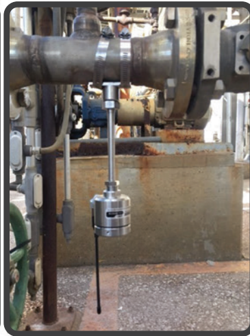
Dual-element unit installed using bands.
