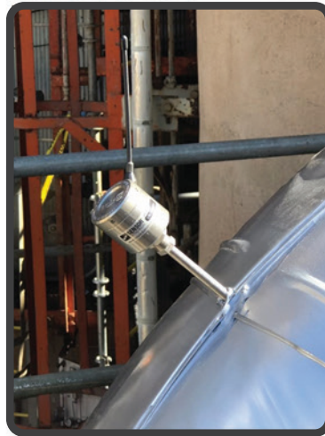
High-temp dual-element unit installed under insulation.
